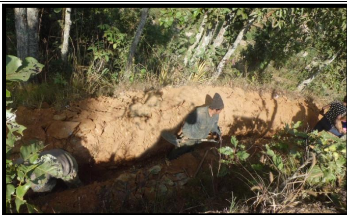
Photo 4: Pipeline trench of Rolpa WSS implemented by RWSSFDB
