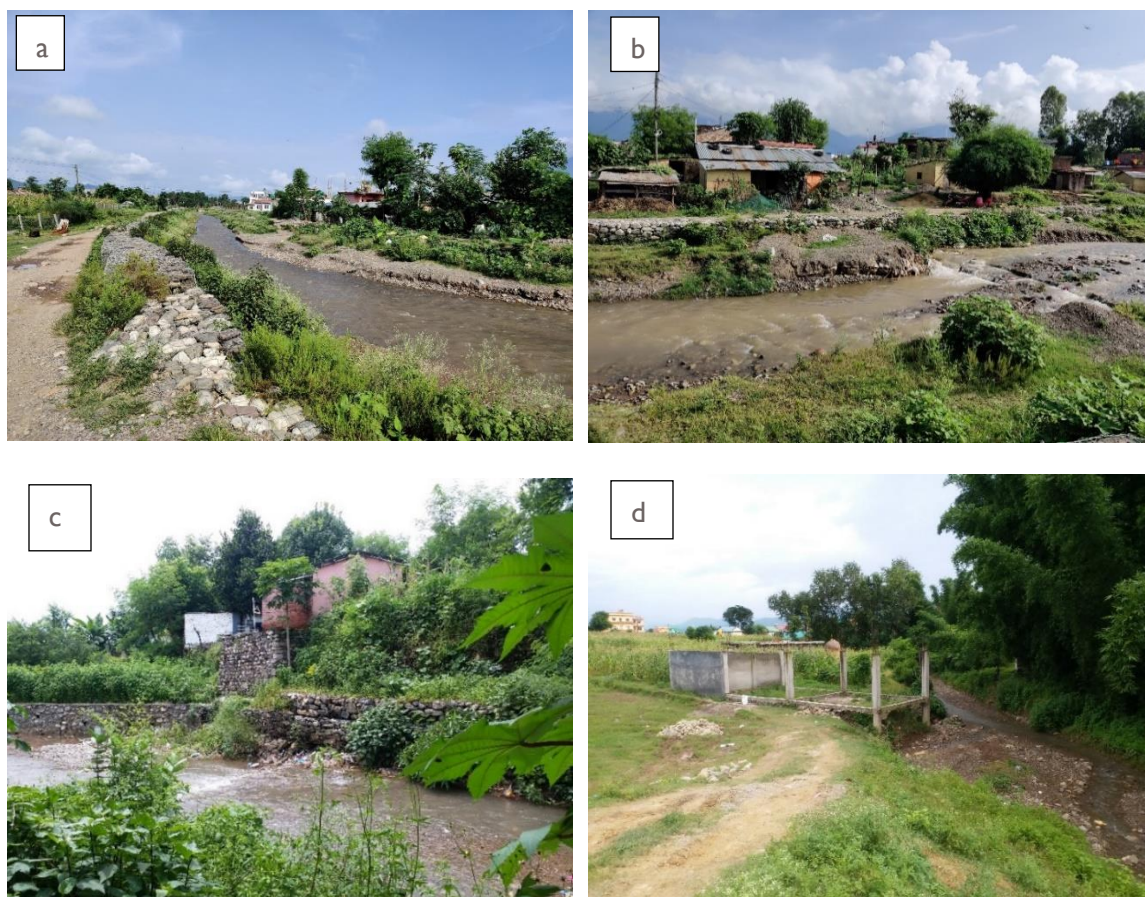
Photograph 0-8: : Severe bank cutting sections of Itaram Khola: a. and b. At the Budbudi village, c. and d. Near to Itaram village
