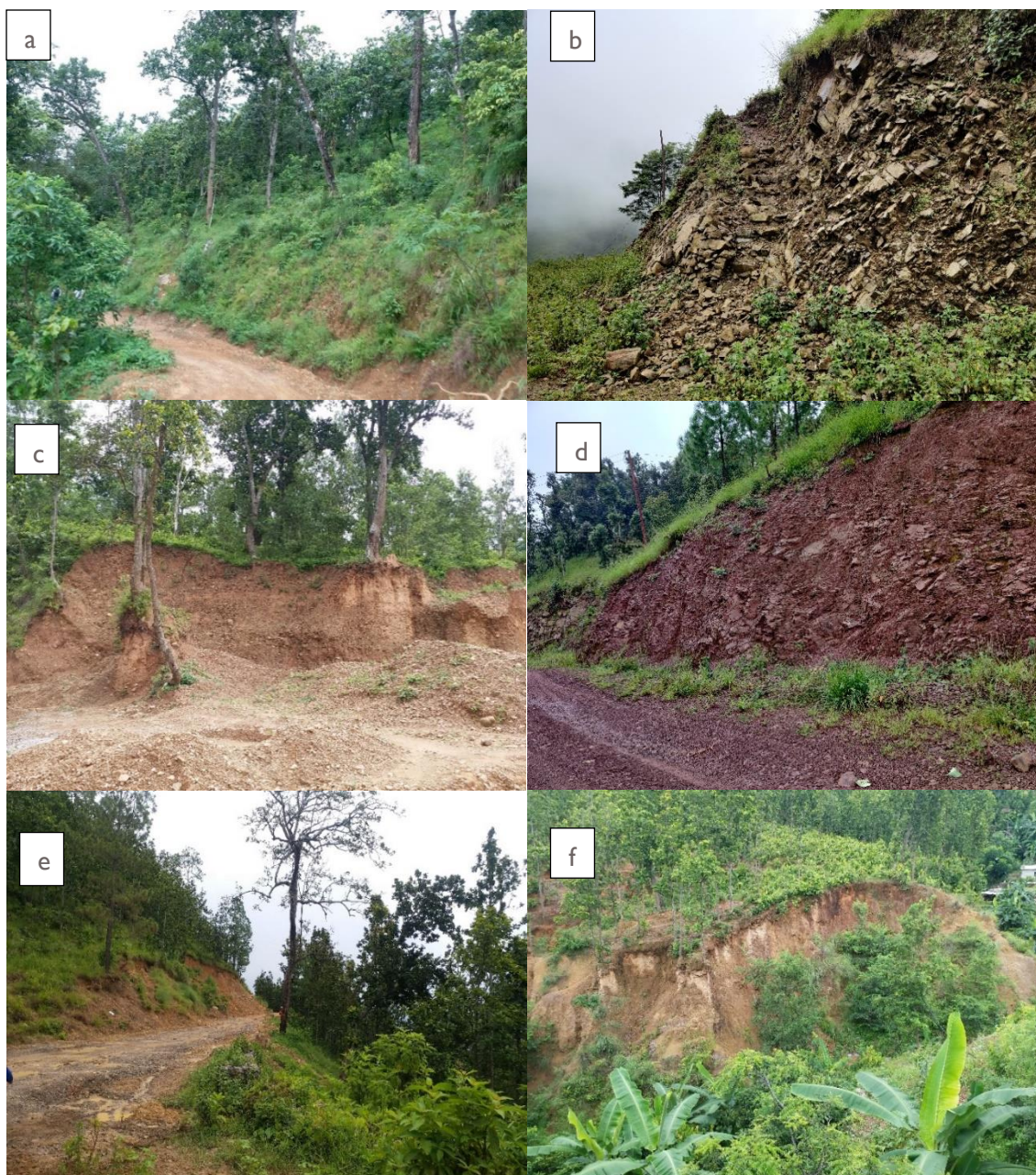
Photograph 0-2: a. weathered quartzite rock, b. Weathered red purple shale, c. and d. Cut slope failures and colluvium soil along Chanabari to Maikal Road, e and f. Excavated alluvial deposits showing potentiality of slides
